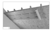
1. Fix the vapour control layer strips horizontally (preferably from top to bottom) or vertically with inscriptions on the inside with pre-installed double-sided tape (e.g. Corotop MIX) or, if the situation requires it (e.g. timber frame), with a stapler. Cover the places where the vapour control layer is perforated by staples with adhesive tape (e.g. Corotop FIX).
