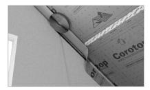
3. The places where the vapour control layer connects to the wall should be sealed with special adhesive or butyl tape (e.g. Corotop BUTYL). It is recommended to use an additional hold down strip and to leave about 2 cm of excess foil (folds).
